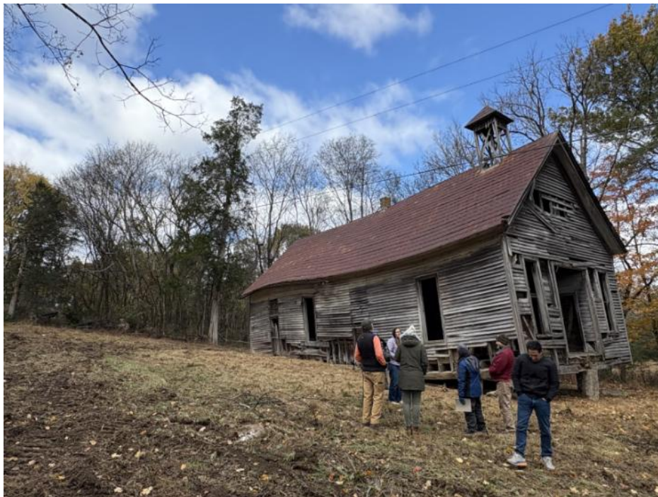
Figure 14: A wider view of the southeast oblique.
