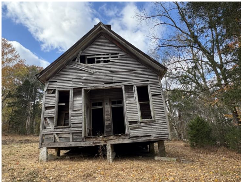
Figure 12: East (front) elevation of Sanders Grove School. Note the symmetrical front and piers raising it from the ground but lack of stairs to the entrance.
