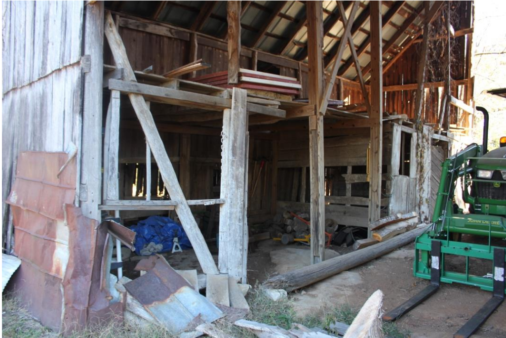
Flanking cribs with missing boards and hay lofts in the barn.
