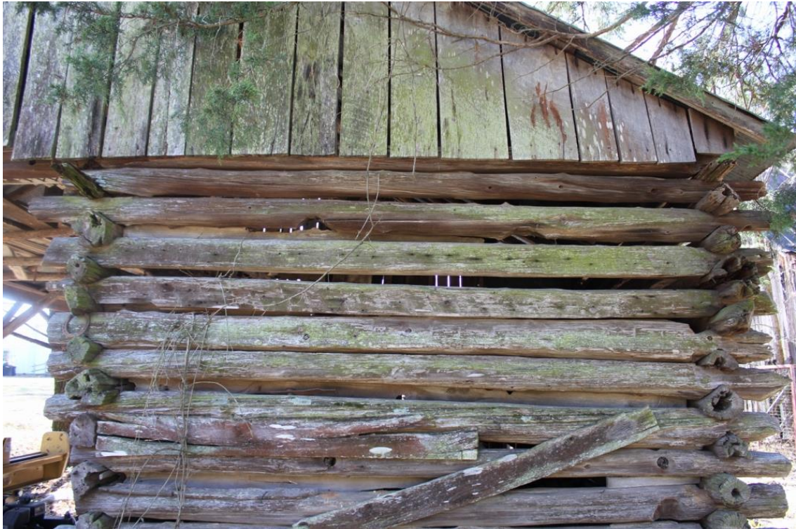
Seen above is the chink construction and different sizes of the timber used on the north side of the corn crib.
