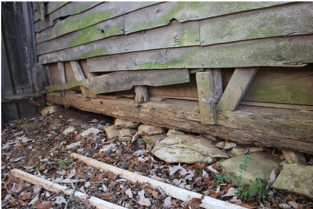
The low, dry-stacked stone foundation beneath the smokehouse.
